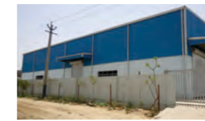
10,000 Sq. Ft. Warehouse at Dharuheda (GGN), For GKN
